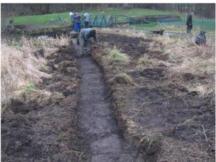
Time was ticking over now and a decision was taken to pull up the diggers and to concentrate on tidying up the site until next time. Some of the excavation spoil was used to back fill the copings on the previously cleared bank the other side of the locks and the rest was raked and spread out to even off the rough areas created by the dig.
